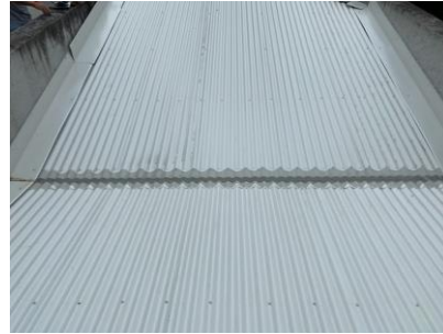
Photos of roofing progress
